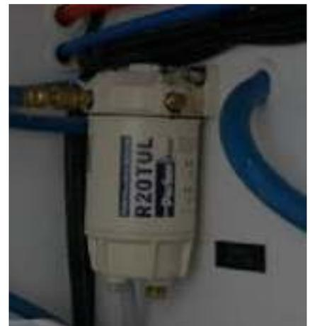
*GENERATOR FUEL PRE-FILTER is behind the generator against the bulkhead*
